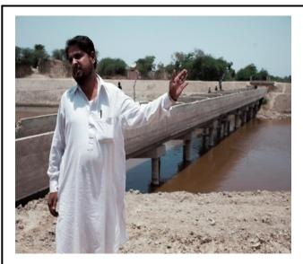
"In the rains of last year this LBOD embankment broke down. This year they have started construction but it is not going very well. The embankment we are standing on should have been 5 feet higher plus this other embankment should have also been 5 feet higher. Instead they have left it incomplete saying it is complete. You can see its condition; if water hits it again it will surely break through the wall.
